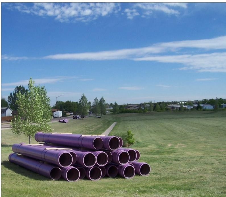
*Above: Purple pipe. The recycled water system includes a separate distribution system for recycled water. To differentiate this system from the potable system, purple pipe was used.*
