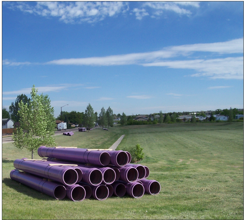
Above: Purple pipe. The recycled water system includes a separate distribution system for recycled water. To differentiate this system from the potable system, purple pipe was used.
