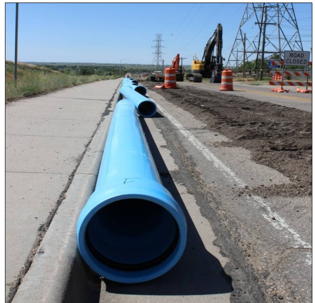
Construction crews prepare to install a 12-inch water main in Walterscheid Boulevard.
