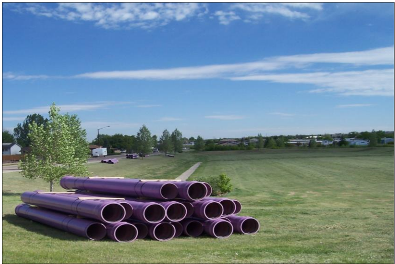
Above: Purple pipe. The recycled water system includes a separate distribution system for recycled water. To differentiate
