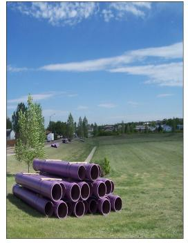
Above: Purple pipe. The recycled water system includes a separate distribution system for recycled water.
