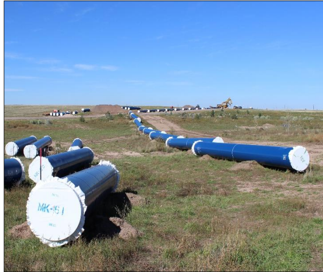
Above: Construction of the Southern Water Transmission Main Phase II.
