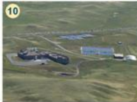
Sherard Water Treatment Plant (Operation 2002 - Present)
