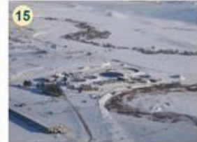
Crow Creek Water Reclamation Facility (Constructed late 1940's - Recycle abilities added in 2007)
