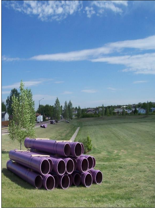
Above: Purple pipe. The recycled water system includes a separate distribution system for recycled water.
