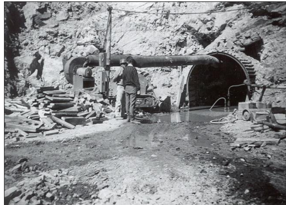
Above: Construction of the Hog Park Tunnel.
