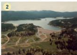
Hog Park Dam & Reservoir (Constructed 1966 & Enlarged 1985)
