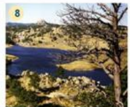
North Crow Dam & Reservoir (Constructed 1911 Rehab in 1994)
