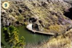
Upper North Crow Dam & Reservoir (Constructed 1930 - Rehab in 1994)
