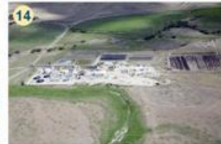
Dry Creek Water Reclamation Facility (Constructed early 1970's - Expanded late 1980's and 2007)
