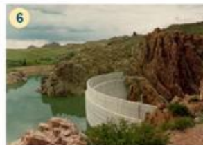
Crystal Lake Dam & Reservoir (Constructed 1909-1910 Rehab in 1986)
