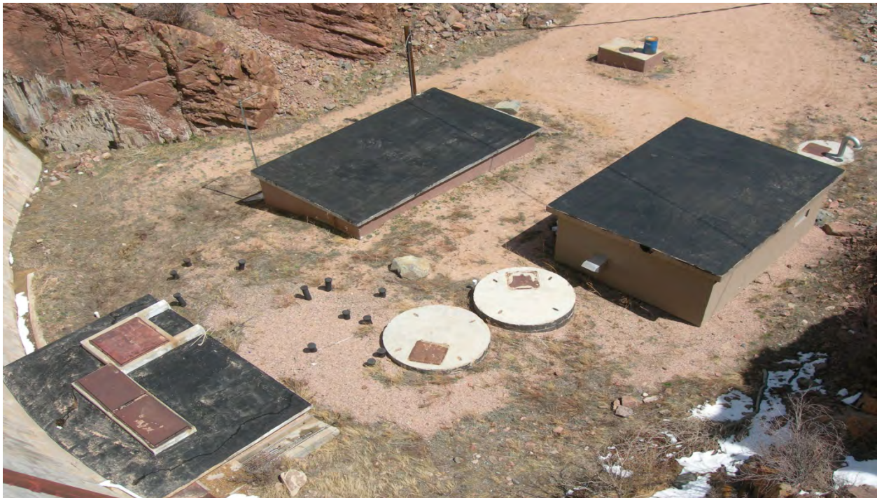
Photo 30: Outlet works buildings. 30" and 50" pipes carry water to a water treatment plant downstream.
