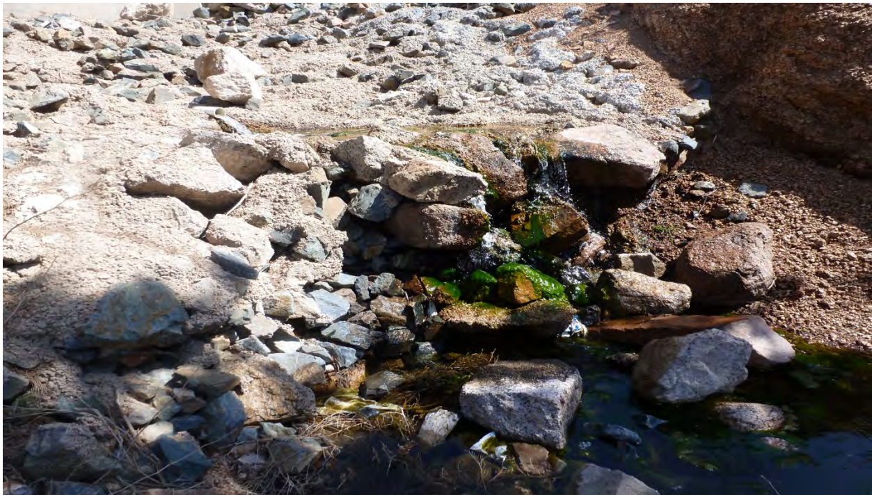
Photo 12: Downstream of grouted riprap below spillway. (May 6, 2013)
