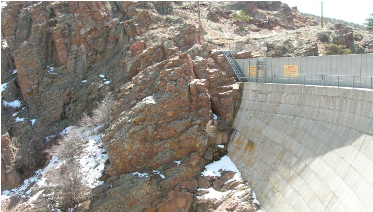
Photo 20: Right abutment. (May 6, 2013)
