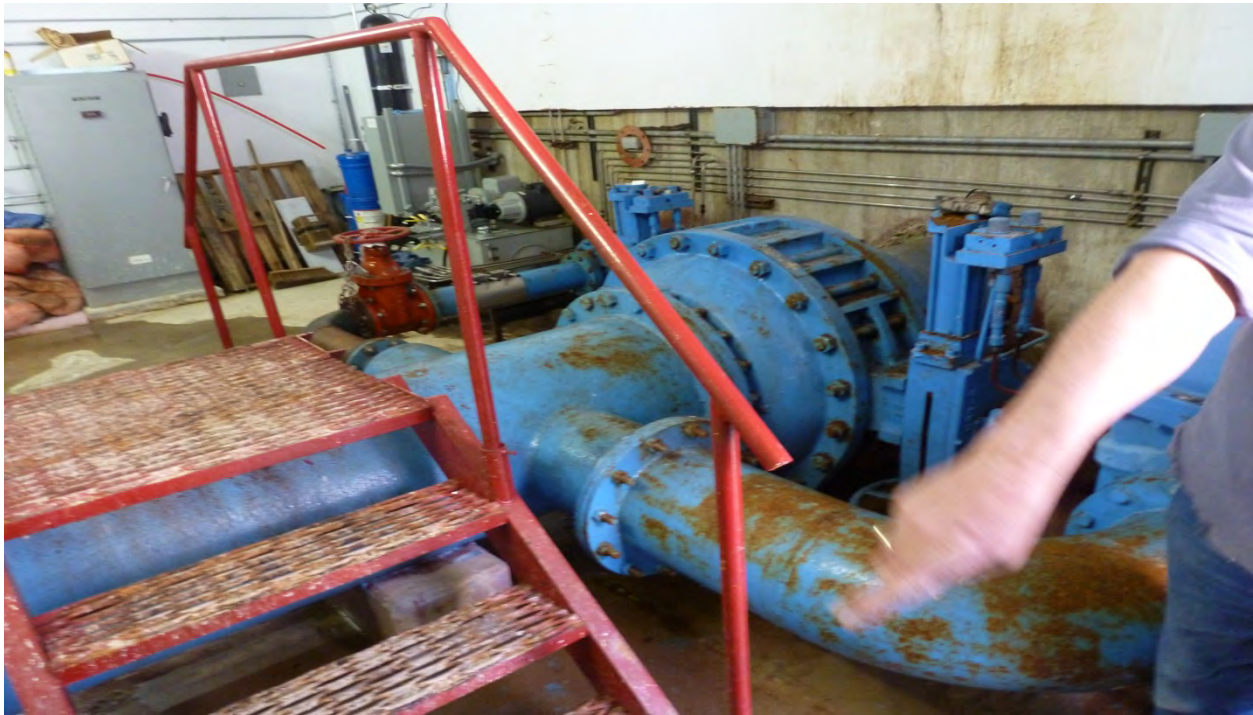
Photo 33: Inside of outlet works building. (May 6, 2013)
