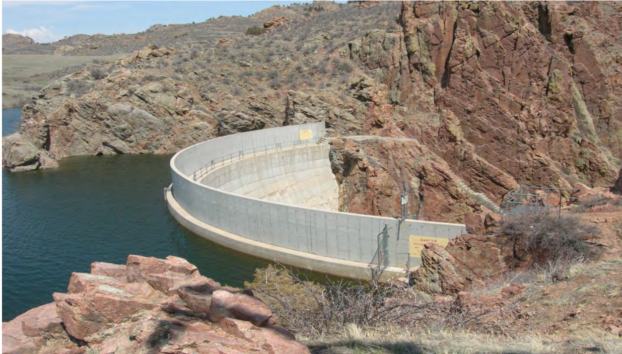
Photo 15: Crystal Lake Dam. (May 6, 2013)
