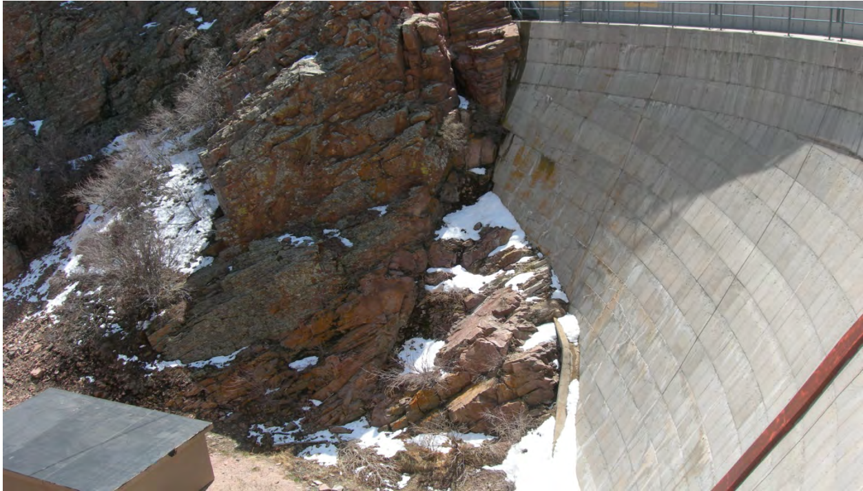
Photo 21: Right abutment. (May 6, 2013)
