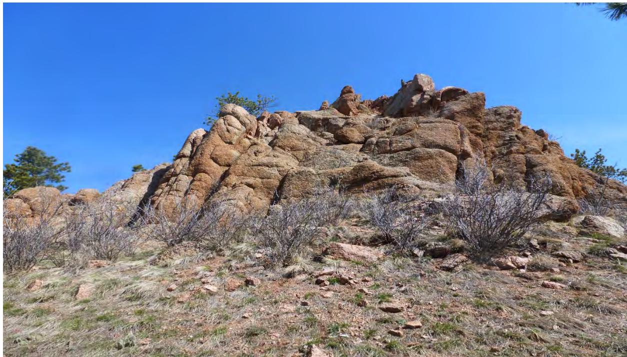
Photo 14: Looking upstream between the left abutment of the dam and right abutment of the main spillway. Notice the near vertical orientation of fractures in the rock.
