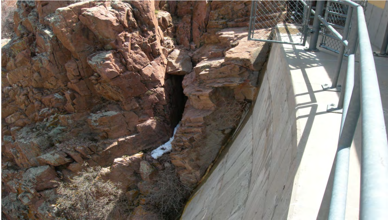
Photo 23: Right abutment. (May 6, 2013)
