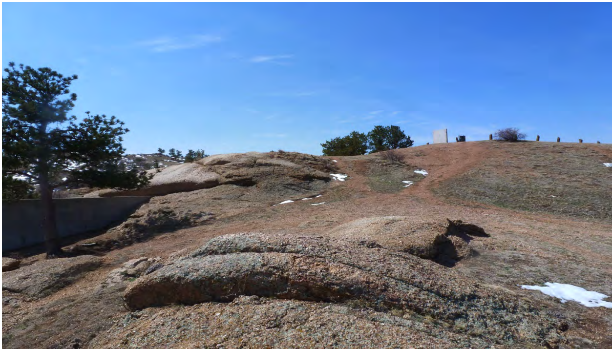
Photo 30: Upstream of right abutment of dam looking downstream and to the southeast. (May 6, 2013)
