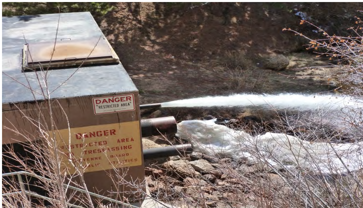
Photo 31: Outlet works outfall pipes. (May 6, 2013)
