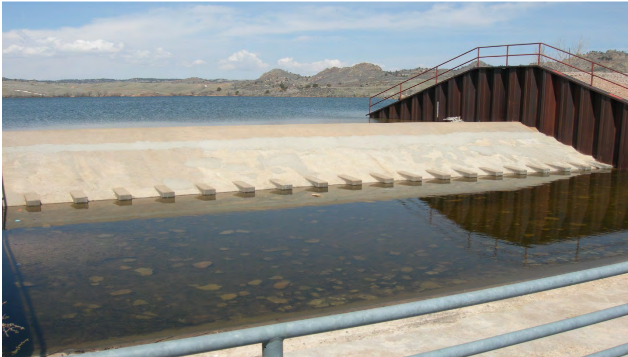
Photo 10: Main spillway looking upstream. (May 6, 2013)
