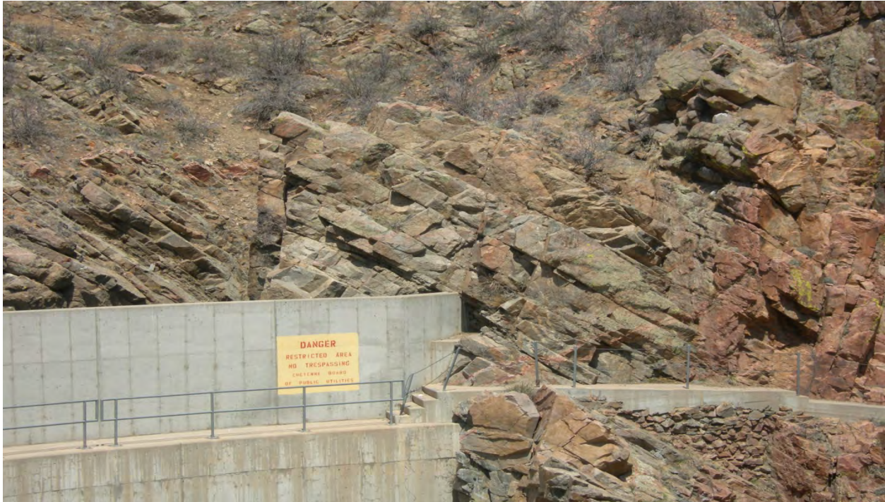
Photo 17: Top of left abutment. Notice the orientation of the rock joints. (May 6, 2013)
