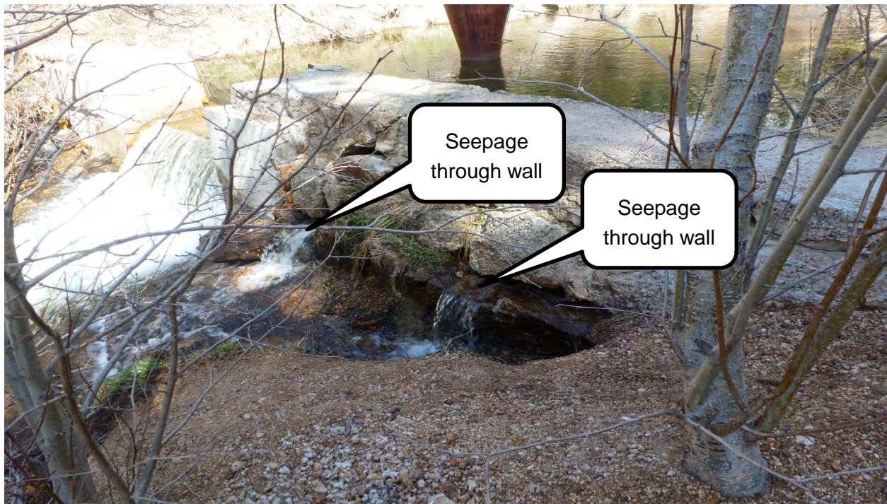
Photo 38: Downstream of weir. Notice water flowing through the wall. Weir measurements will not be accurate. (May 6, 2013)
