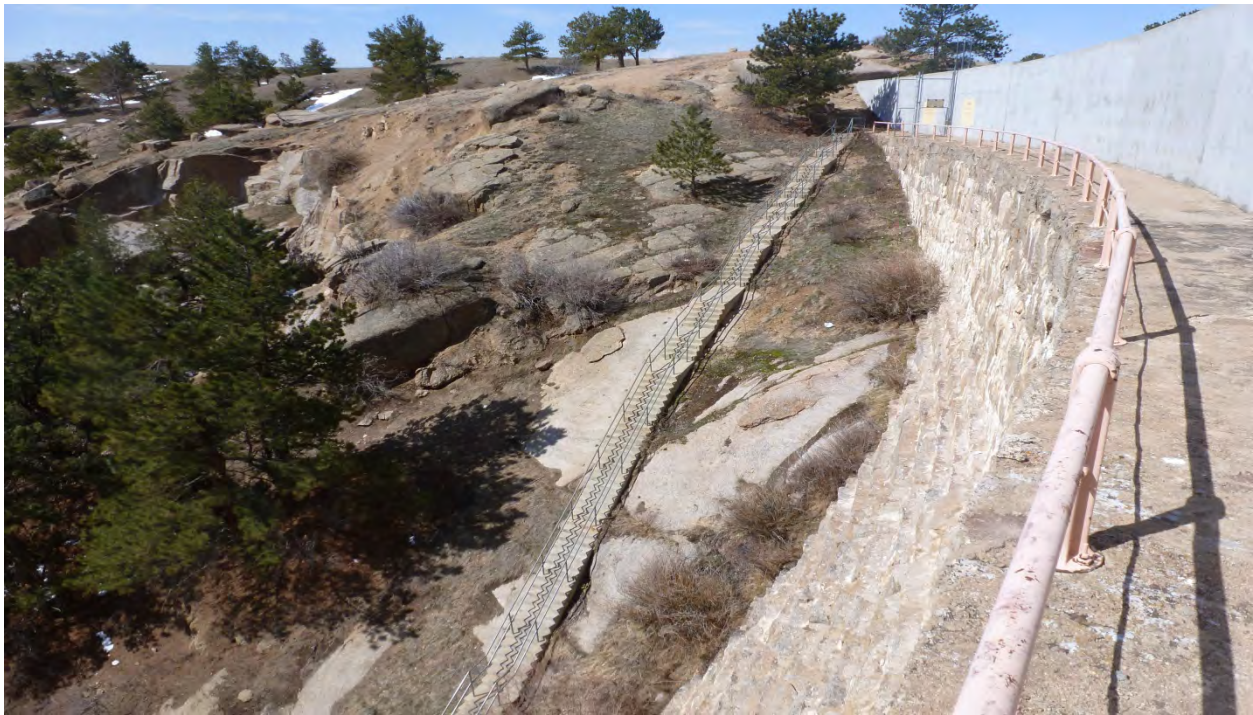
Photo 20: Right abutment of dam. Some shrub growth along abutment. (May 6, 2013)
