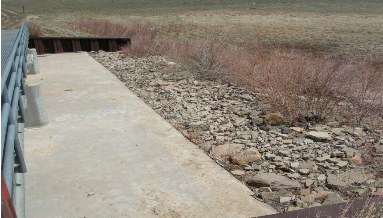
Photo 9: Downstream of main spillway. (May 6, 2013)
