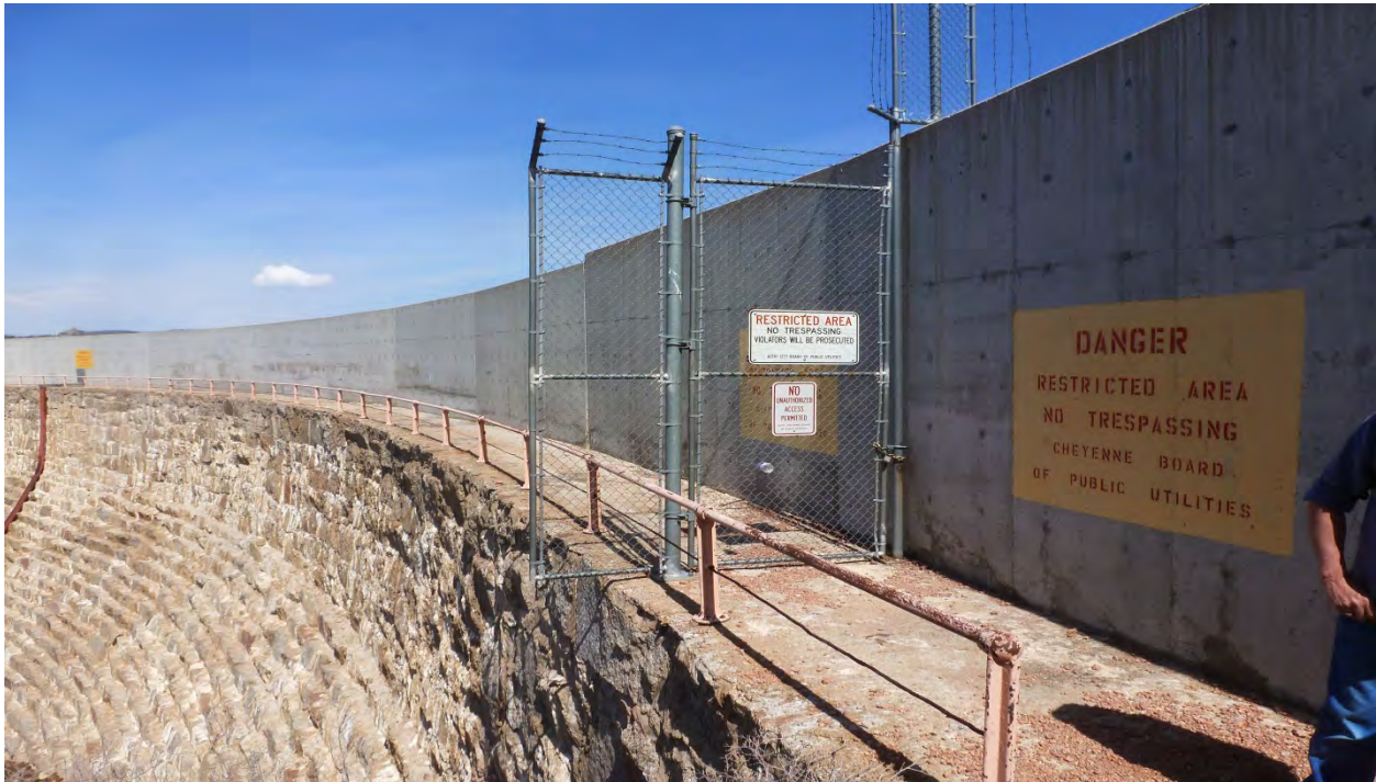
Photo 35: Security gate. Typical both sides. (May 6, 2013)
