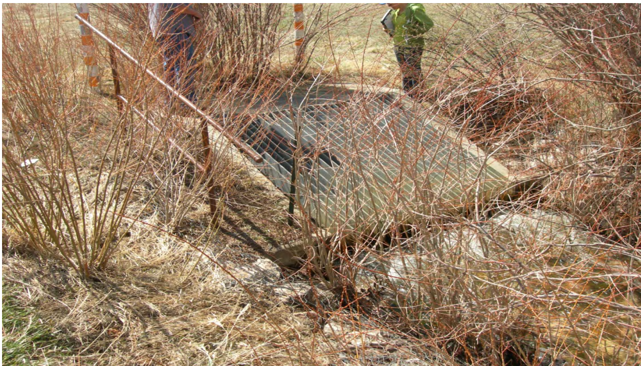
Photo 42: Outfall of pipeline from Lake Owen to Granite Springs Reservoir. (May 6, 2013)
