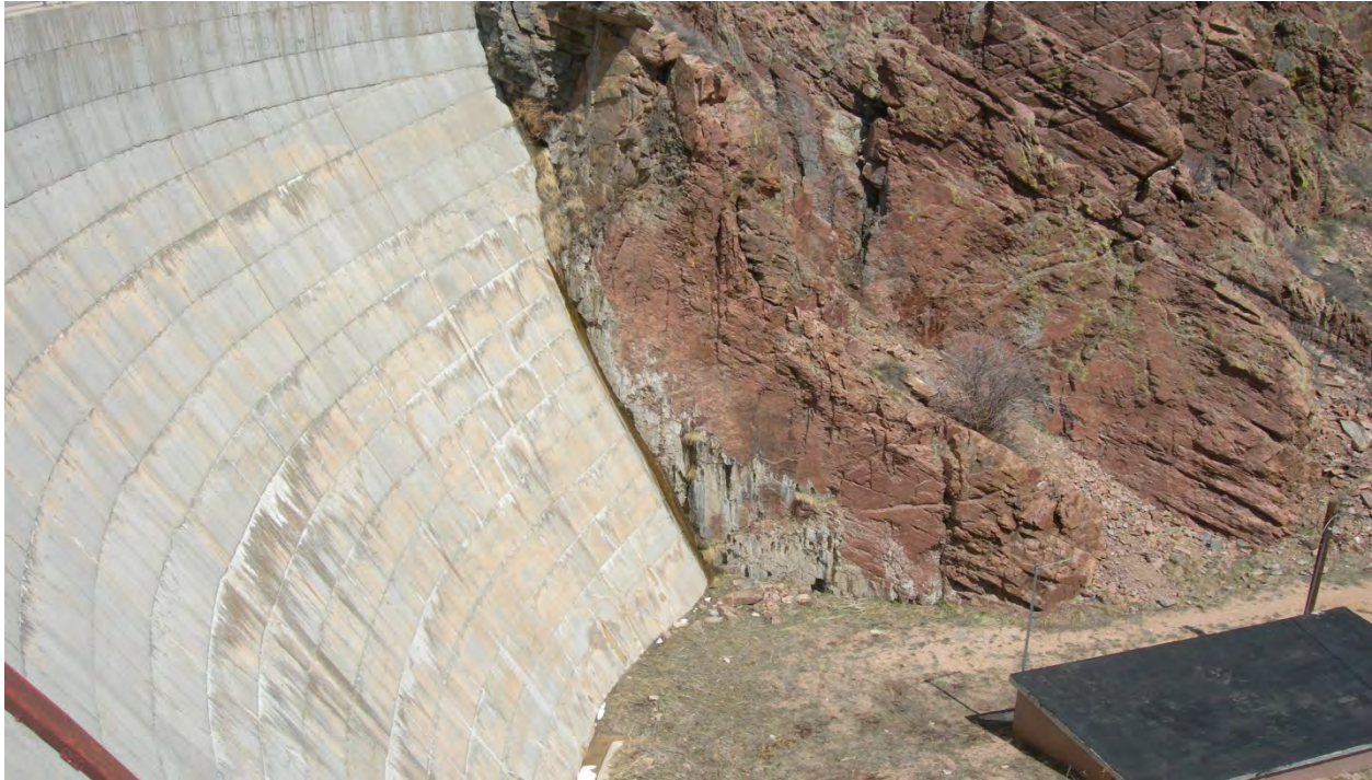
Photo 19: Left abutment and downstream face. (May 6, 2013)
