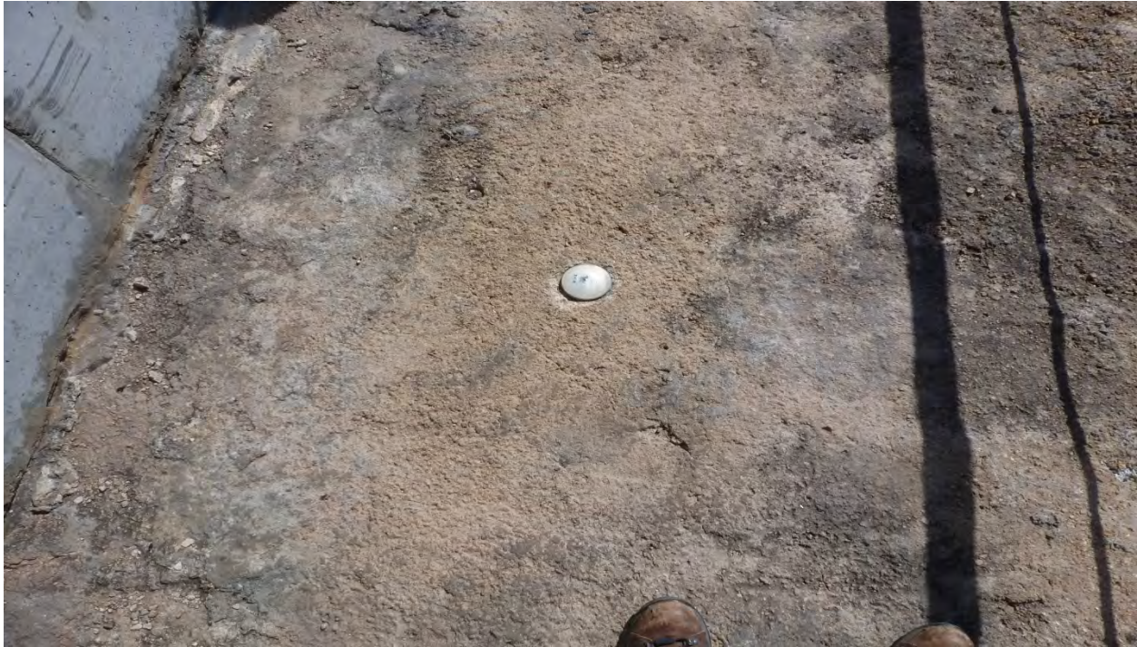
Photo 25: Survey monument marker on dam crest. Three markers total. (May 6, 2013)
