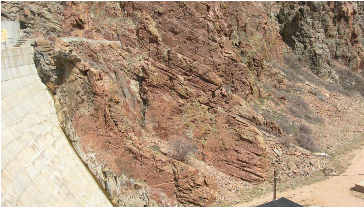
Photo 16: Left abutment. (May 6, 2013)
