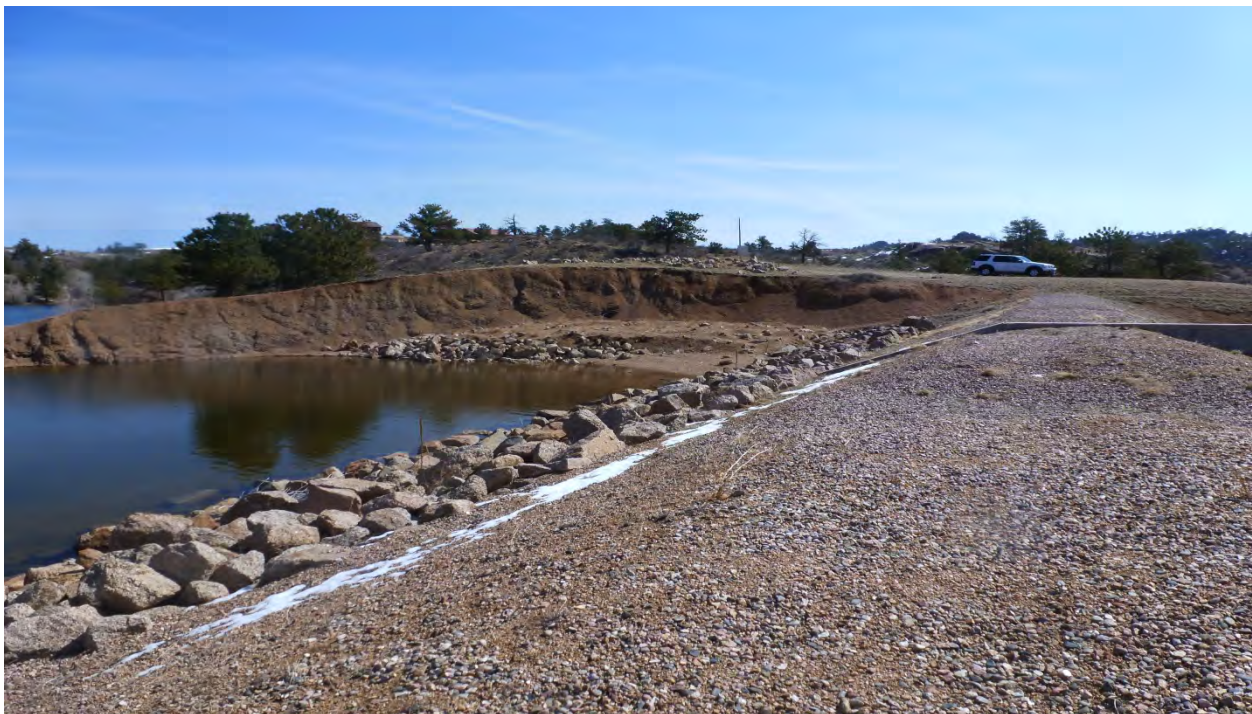
Photo 4: From right-most fuse plug, looking northeast across fuse plugs. (May 6, 2013)
