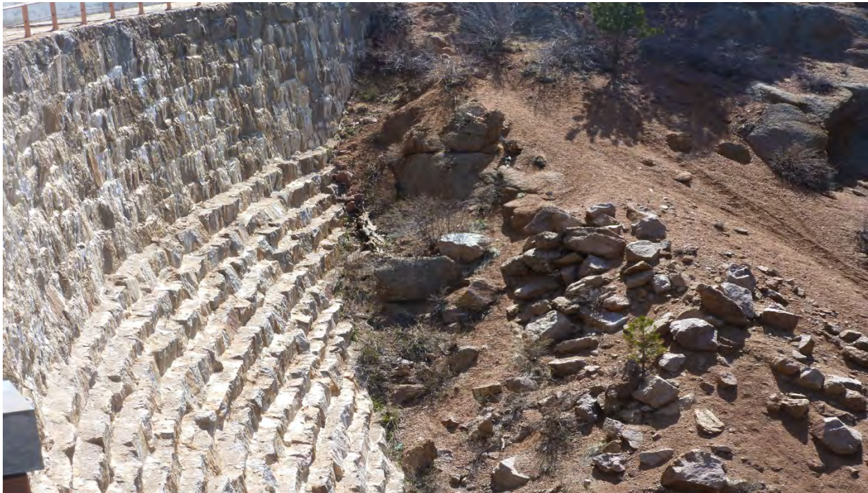
Photo 18: Left abutment of dam. (May 6, 2013)
