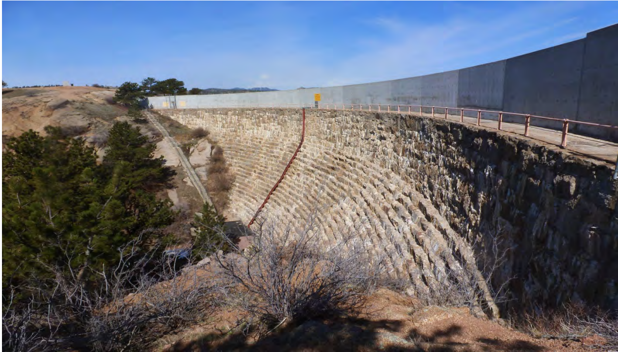
Photo 15: From left abutment, looking west at upstream face of dam.
