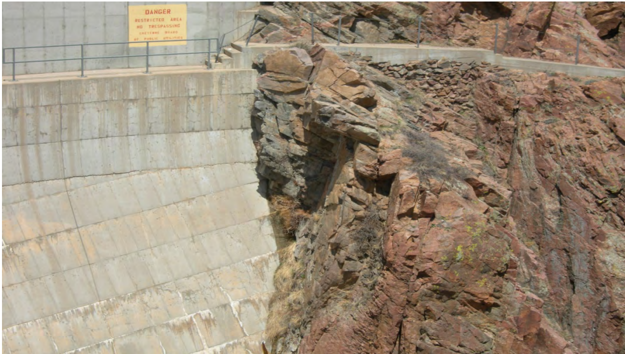
Photo 18: Left abutment. (May 6, 2013)
