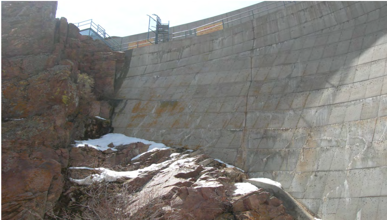
Photo 22: Right abutment and downstream face. (May 6, 2013)
