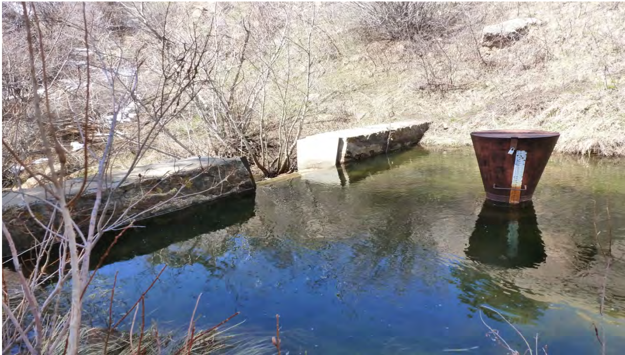
Photo 36: Downstream weir. (May 6, 2013)
