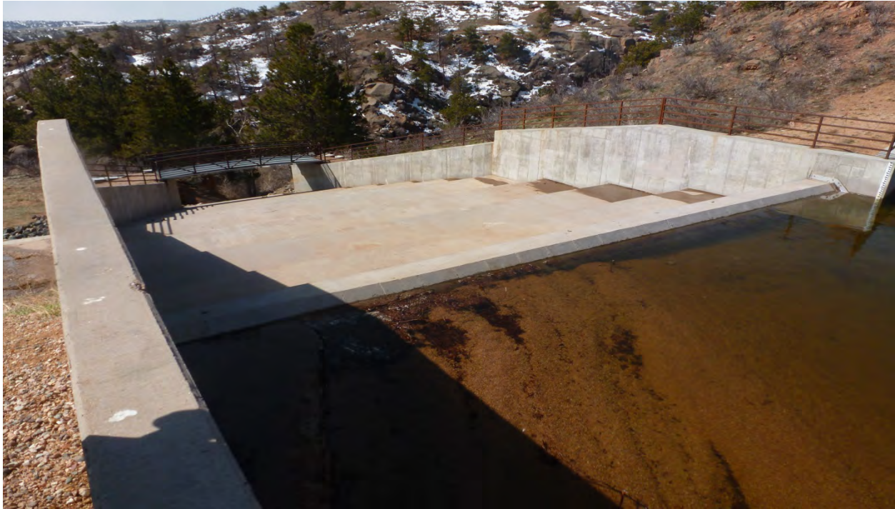
Photo 9: Granite Springs main spillway looking downstream. (May 6, 2013)
