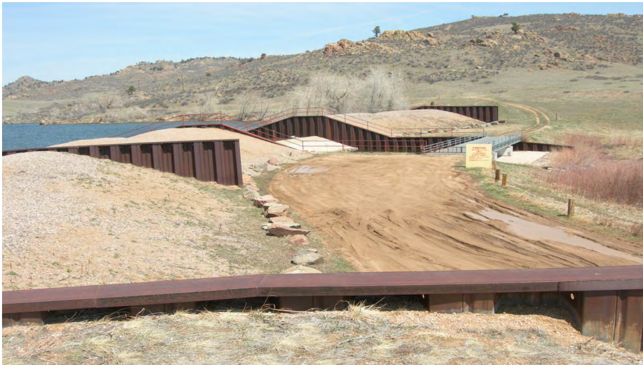
Photo 6: Downstream side of the three fuse plugs and main spillway. (May 6, 2013)
