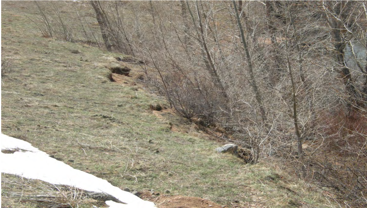
Photo 3: Sloughing of existing ground to the right (south) of the fuse plugs. See Photo 2 for reference. (May 6, 2013)
