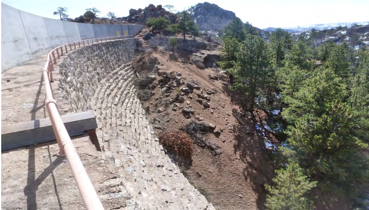
Photo 17: Left abutment of dam. No visible seepage. (May 6, 2013)
