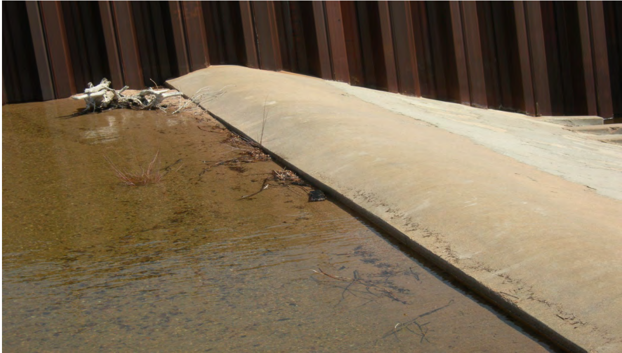
Photo 7: Water level relative to main spillway. (May 6, 2013)
