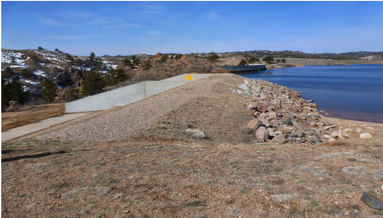
Photo 1: From left abutment of spillway fuse plugs looking west. (May 6, 2013)
